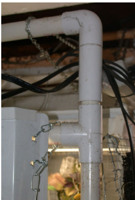
THE UPPER CORNER OF ONE OF THE GATES, SHOWING THE TWO TYPES OF COMMONLY AVAILABLE PVC PIPE JOINTS, AS WELL AS A VERTICALLY-MOUNTED LIGHT FIXTURE.
