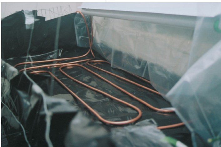
STRATEGICALLY-PLACED COPPER TUBING BENEATH THE WARM-GROWING AREA CIRCULATES HOT WATER TO WARM THE ORCHIDS ABOVE.
